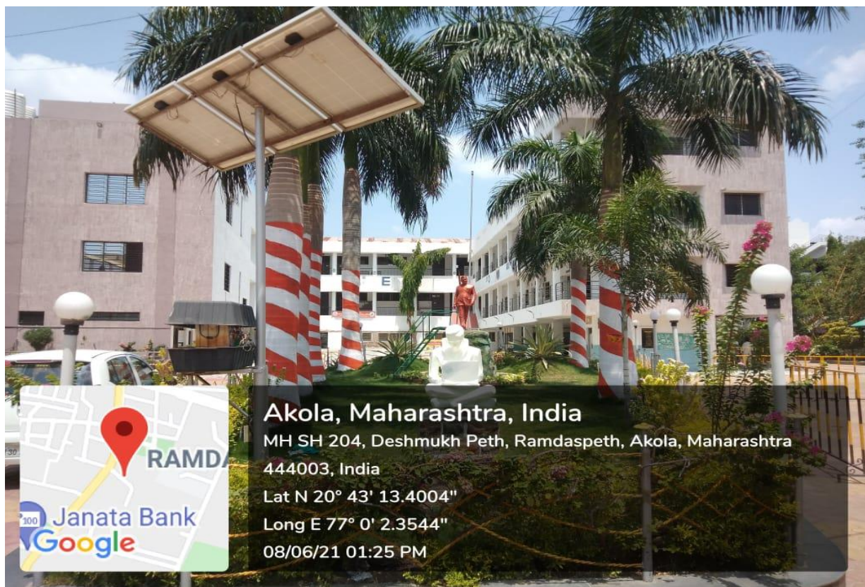
Solar Panel base lights and fountain
